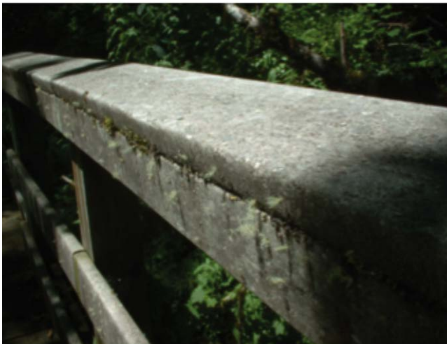
Figure 5: Guard rail in Oregon with fungal fruiting bodies growing on it.
